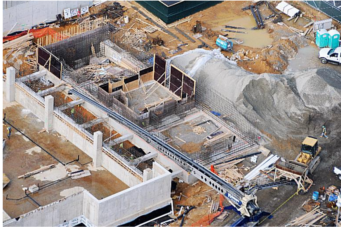
Construction of the mass concrete linear accelerator vaults
